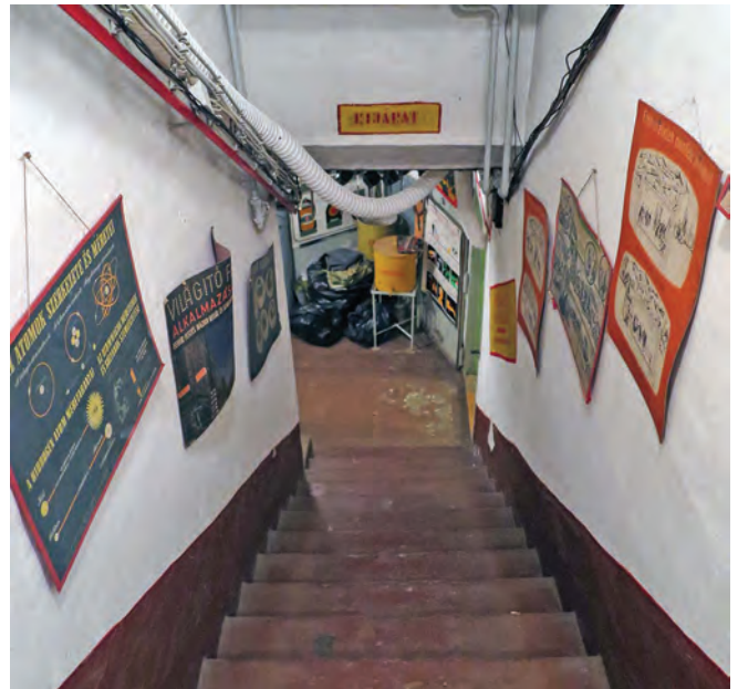
Stairway to the upper level in Csepel shelter number 2 ventilation system. The options seemed to be to suffocate or be roasted.
